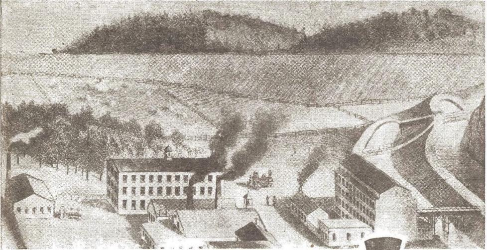
**FIRM** of Rogers, Ketchum & Grosvenor occupied old "Jefferson Works." Two raceways providing water power are at the right with the high embankment of the Morris Canal behind them
