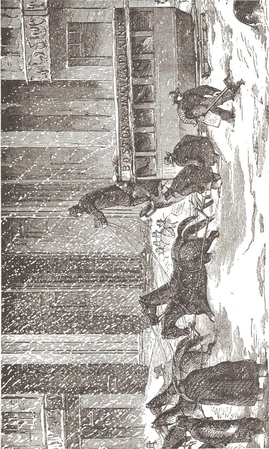
**WINTER STREET, BOSTON, IN 1857.** When heavy snow covered the tracks, some cars were converted into sleighs, their wheels being removed and bodies mounted on runners
